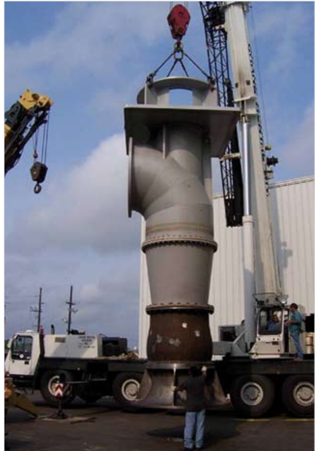
Circulating water pump
