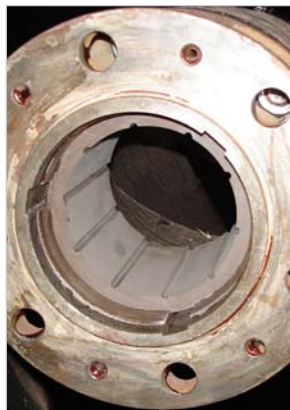
AR1 in center of shaft construction
